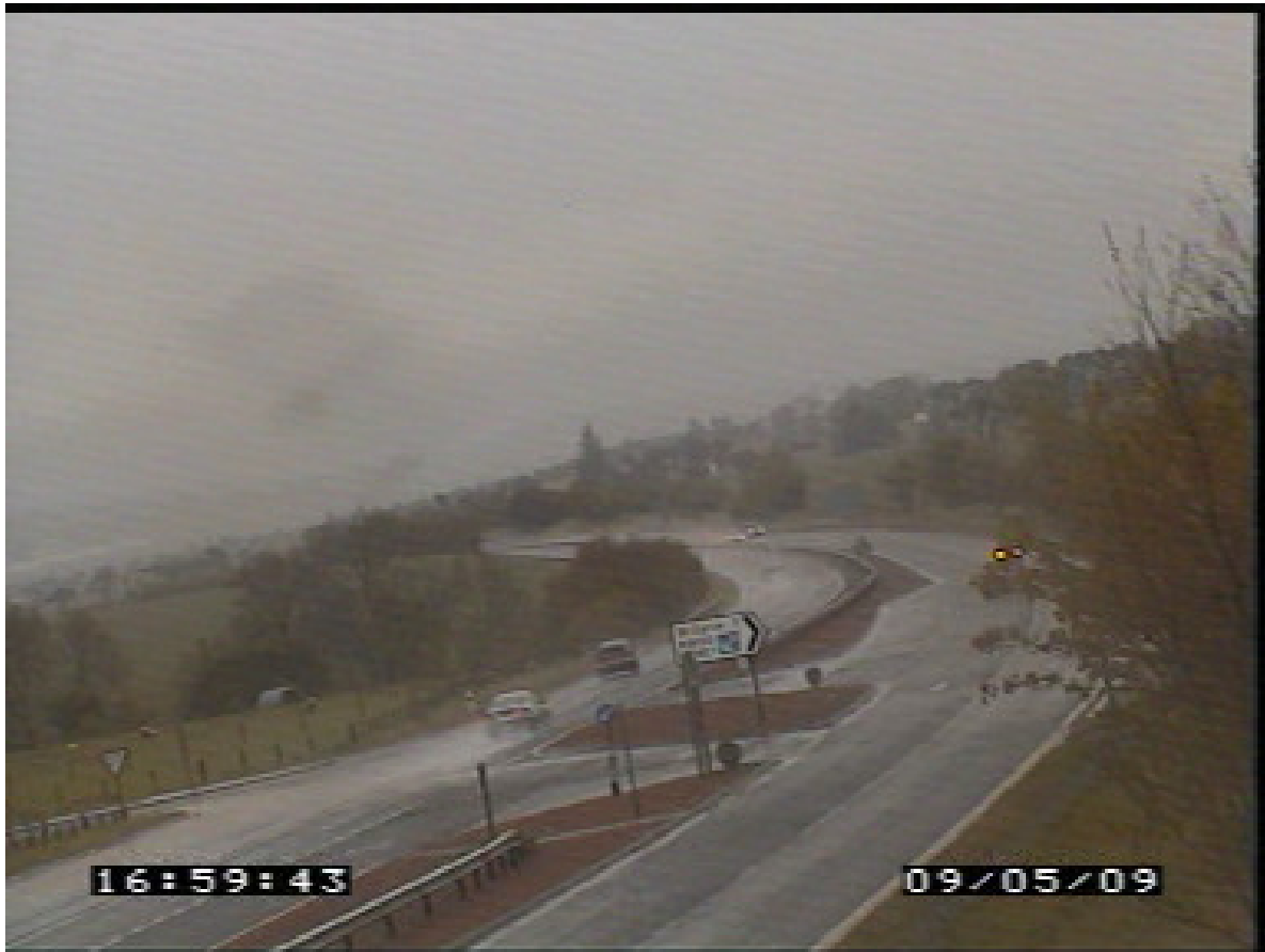
Picture 7.2 Example of Predominant Conflict at the A90/B9120 Junction involving A90 Northbound Traffic Braking and Changing Lanes to Accommodate Left-turners from Laurencekirk
