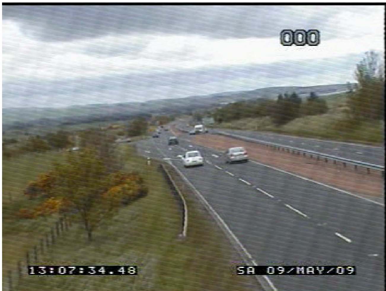
Picture 7.3 Example of Predominant Conflict at the A90/A937 North Junction involving A90 Northbound Traffic Braking and Changing Lanes to Accommodate Left-turners from Laurencekirk
