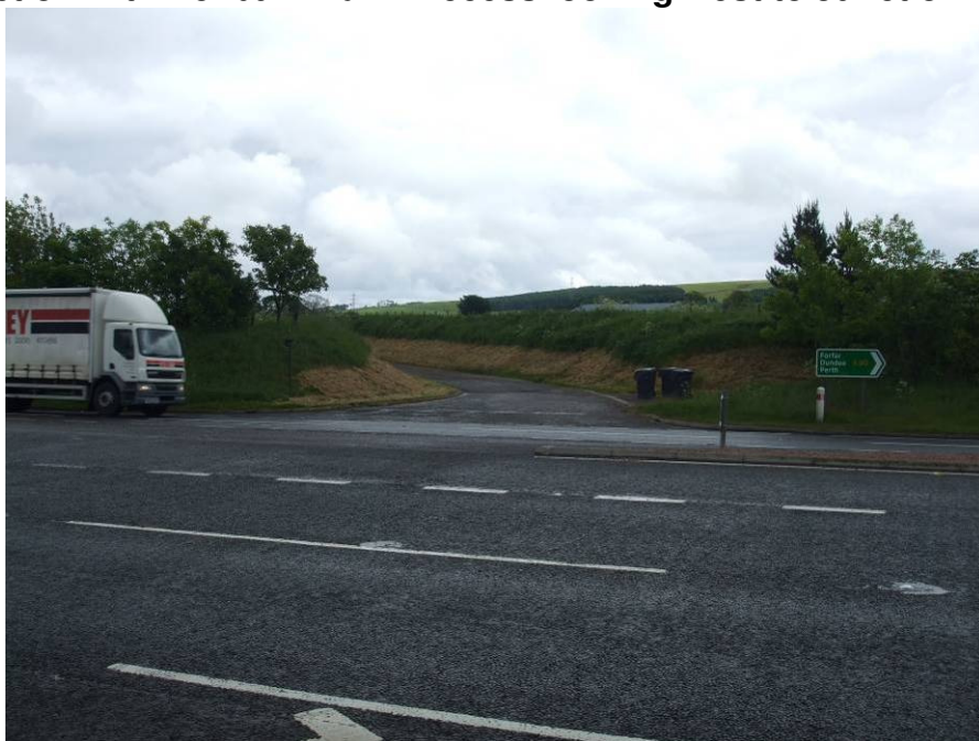
A90 Junction with A937 North – looking east to Keilburn Farm Access
