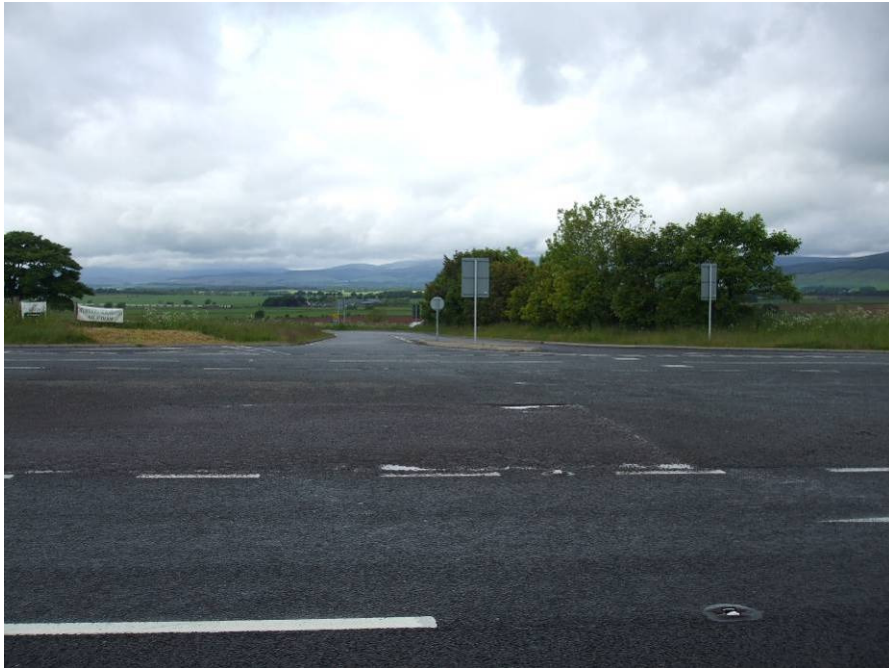
A90 Junction with Keilburn Farm Access looking west to Junction with A937
