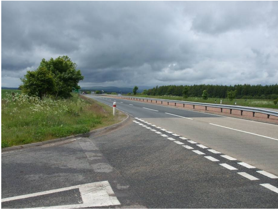
A90 Junction with A937E (South Junction) – looking south
