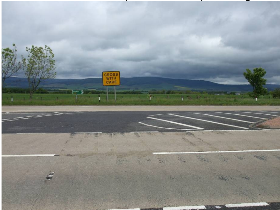
A90 Junction with A937E (South Junction) – looking west
