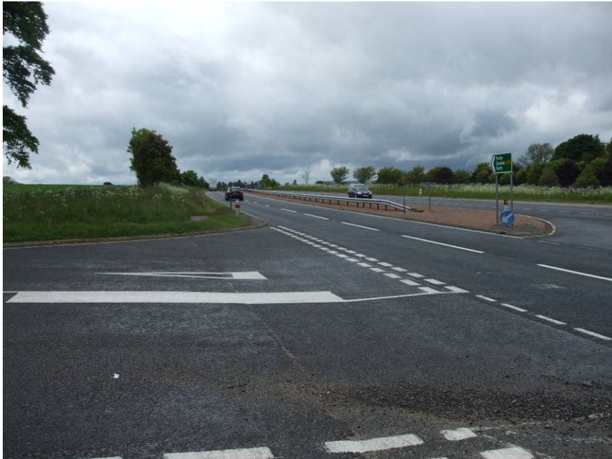
A90 Junction with B9120(E) – looking south
