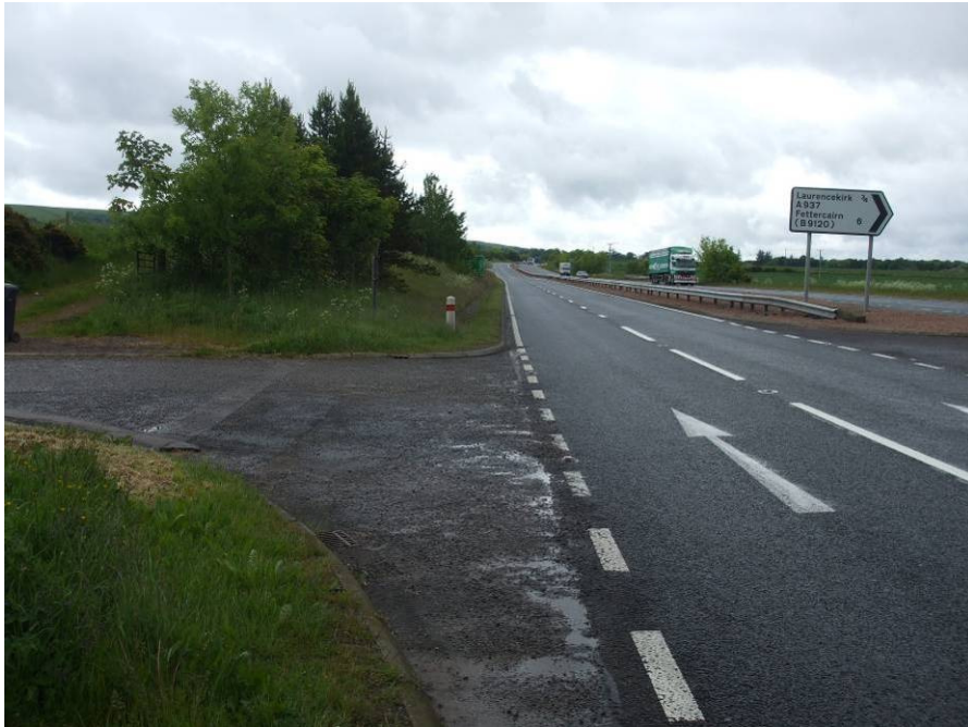
A90 Junction with Keilburn Farm Access – looking south
