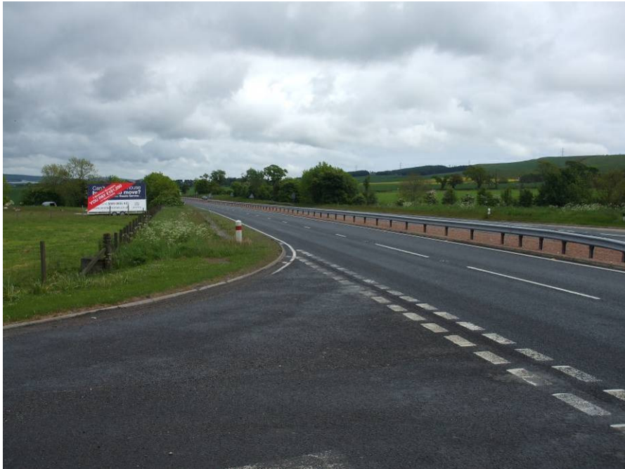
A90 Junction with B9120(W) – looking north
