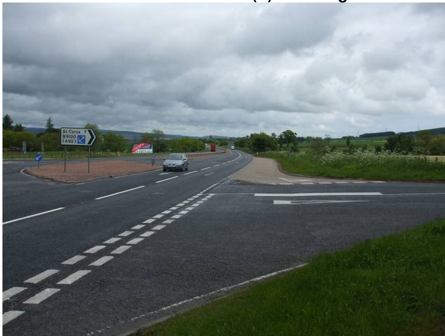
A90 Junction with B9120(E) – looking north
