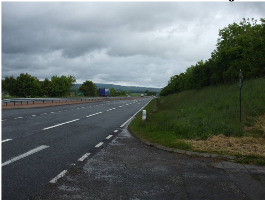
A90 Junction with Keilburn Farm Access - looking north
